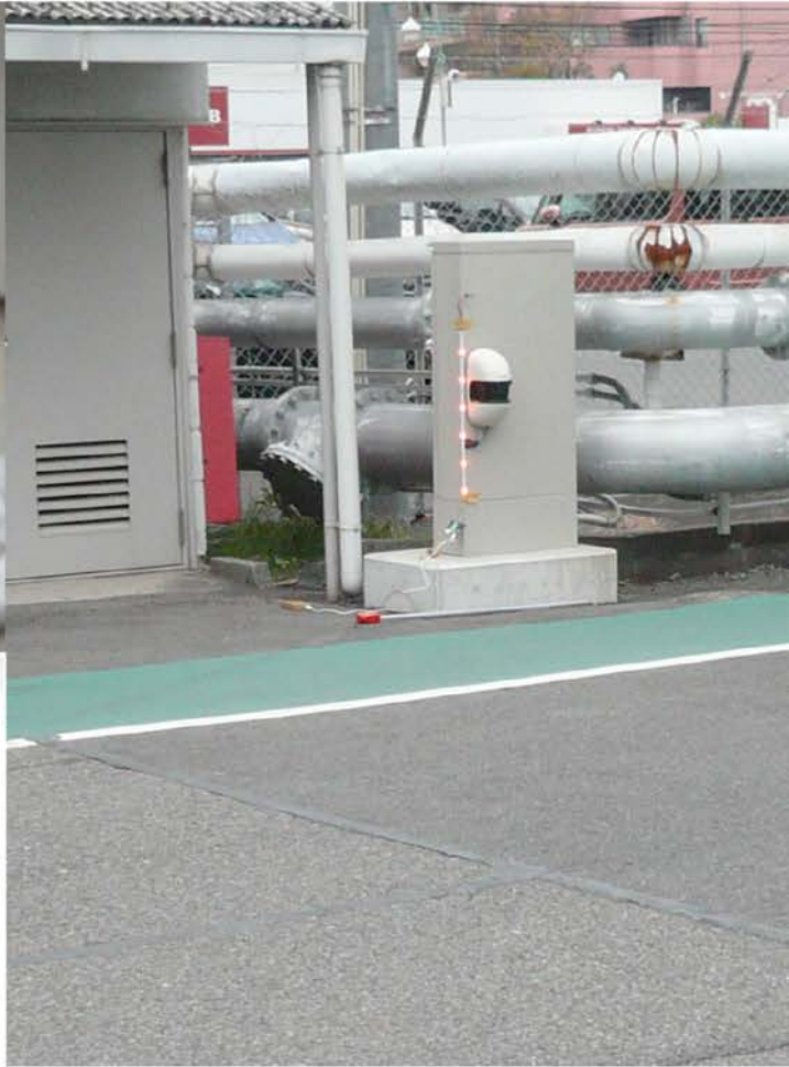
On Field Investigation
